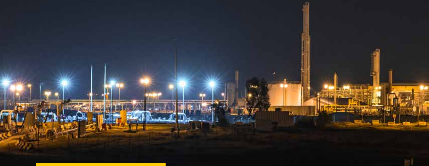
Khor Mor Gas Processing Plant.
