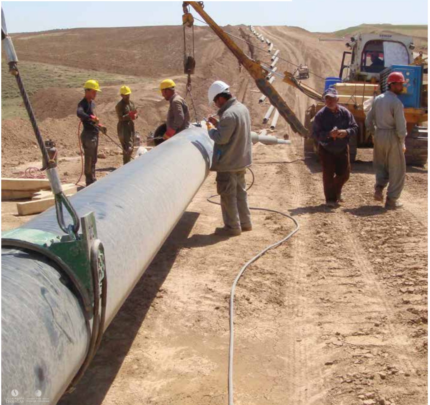
Pipe laying in progress
