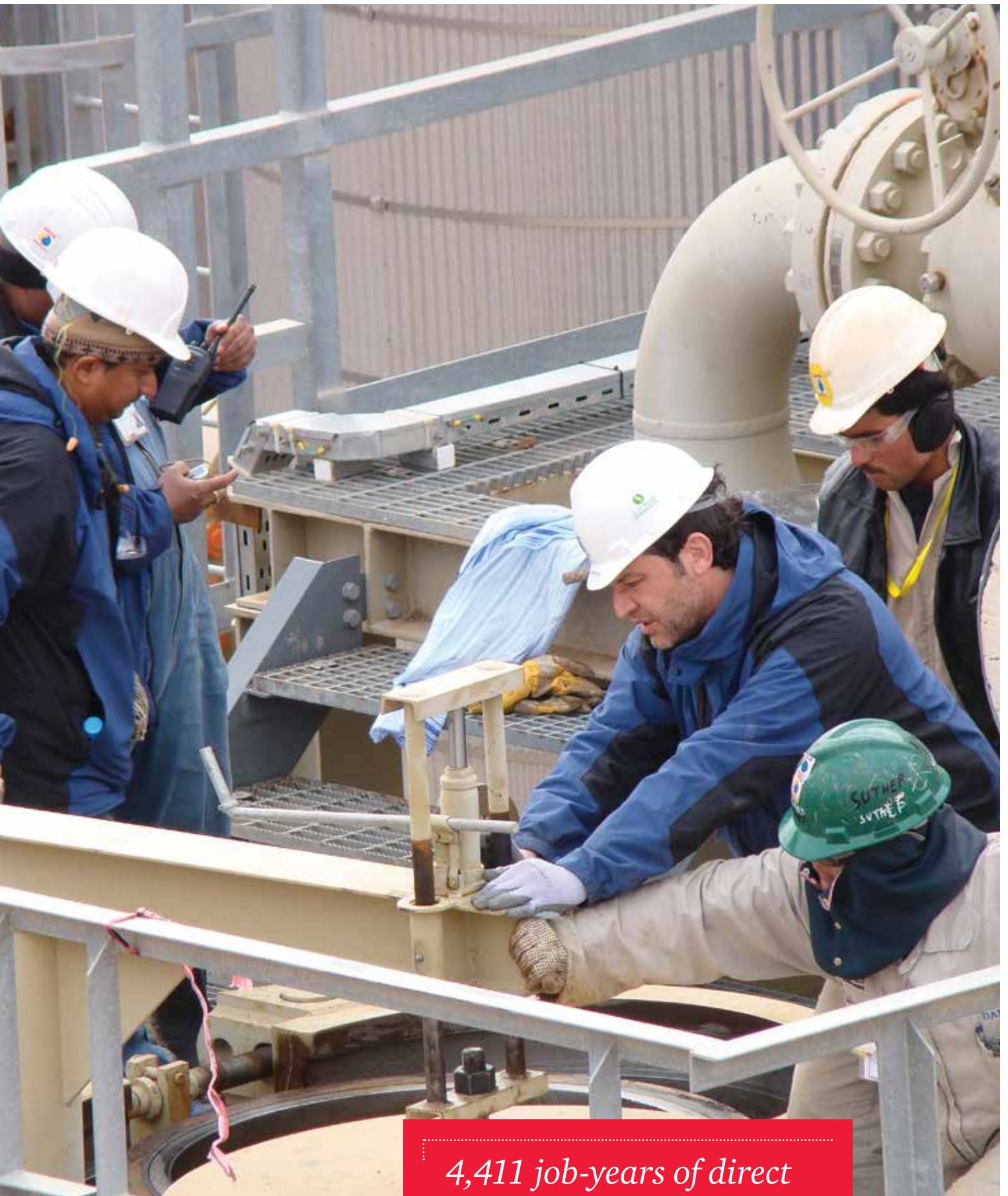
Plant construction work in progress
