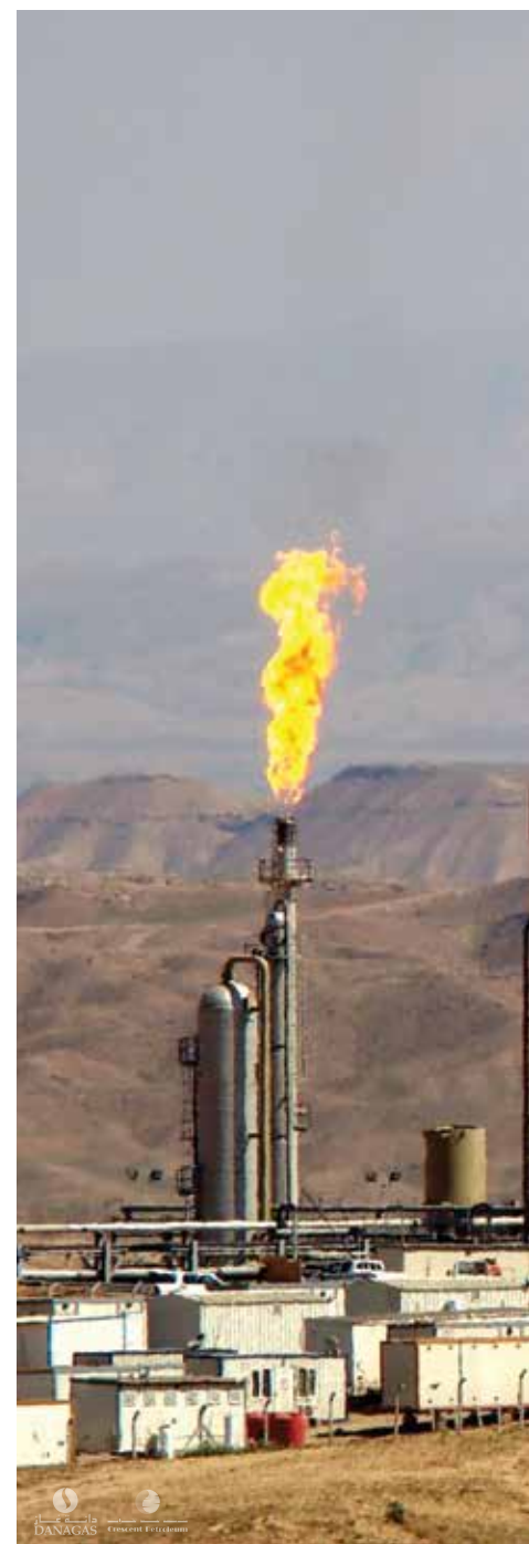
Full view of the plant
