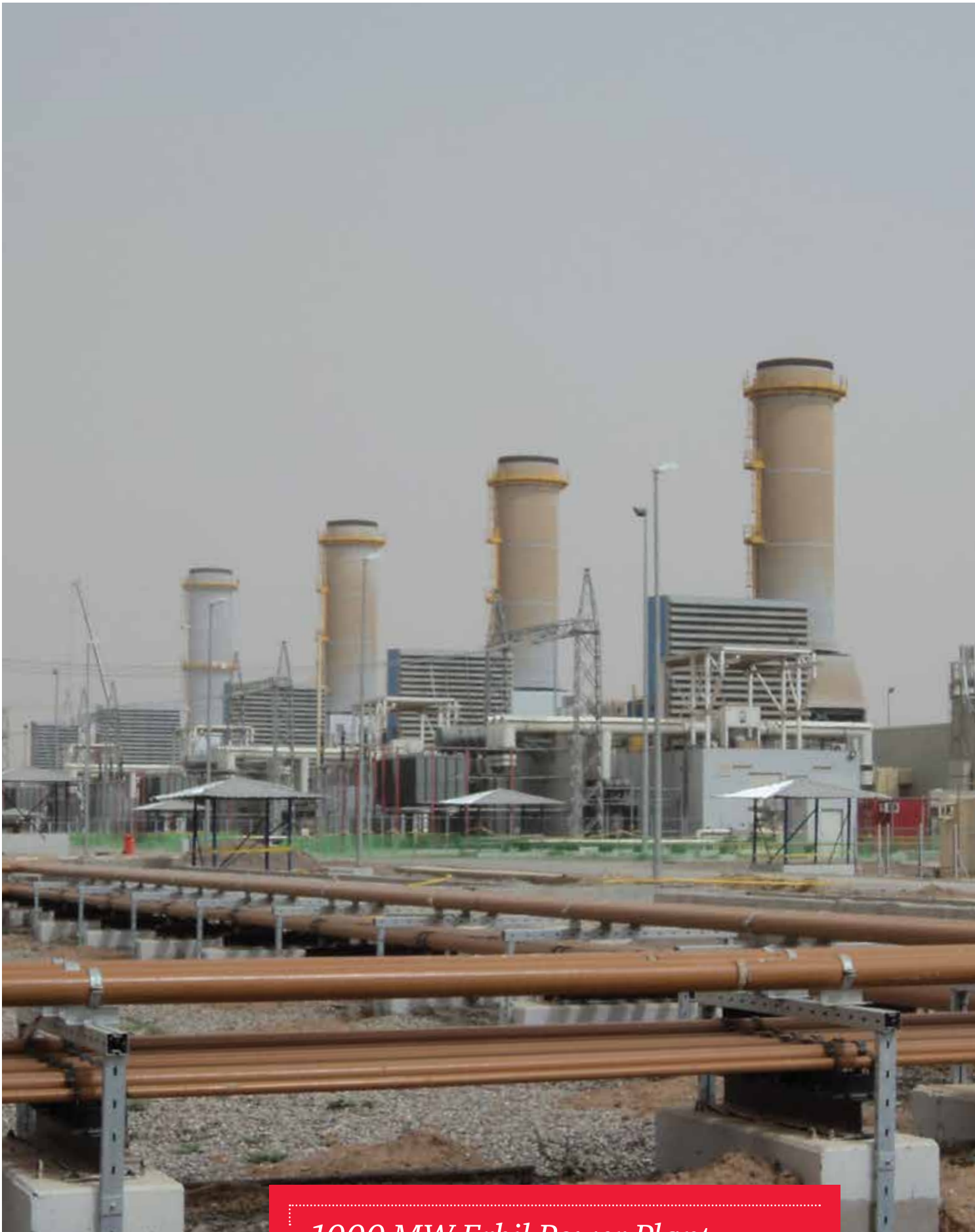
Erbil Power Plant
